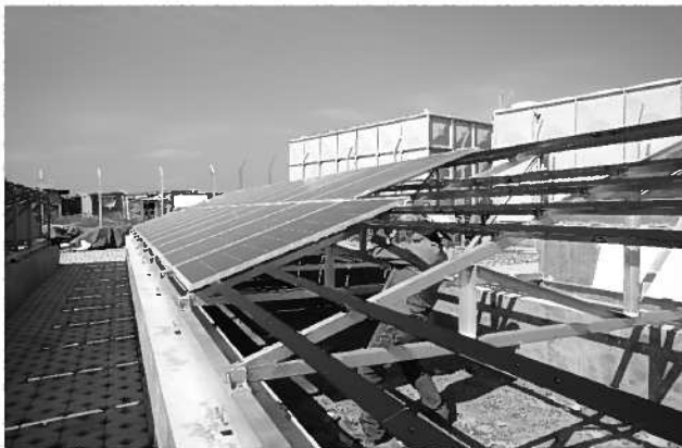
Fig. 4. The foundation and superstructure for the PV supporting frames
