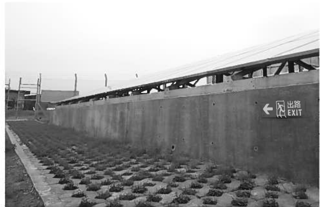
Fig. 5. Precast paving blocks for access and maintenance paths of the PV yard
